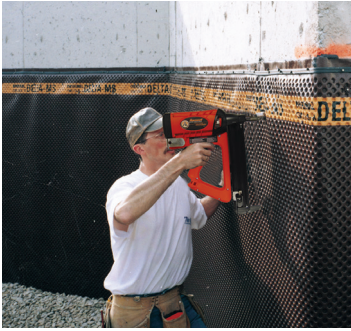
Waterproofing to concrete
