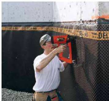
Waterproofing to concrete
