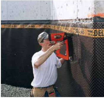
Waterproofing to concrete
