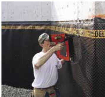
Waterproofing to concrete
