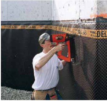
Waterproofing to concrete
