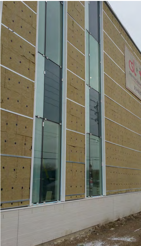
Exterior Walls - Insulation to Steel
