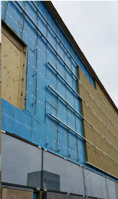
Exterior Walls - Insulation to Concrete
